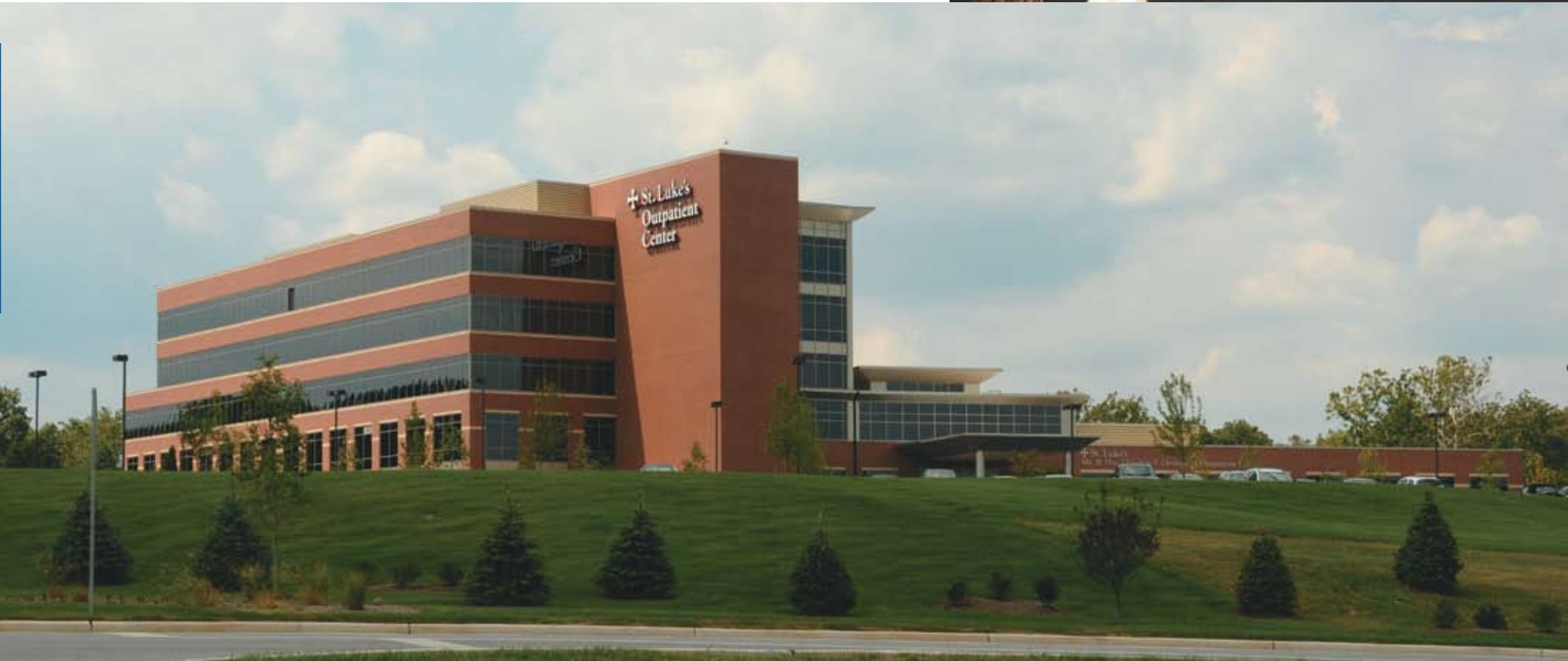
The Mr. and Mrs. Theodore P. Desloge, Jr. Outpatient Center, located directly across from the hospital on the west side of Highway 141.
