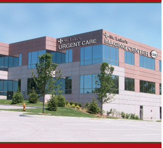
WingHaven® Medical Building
