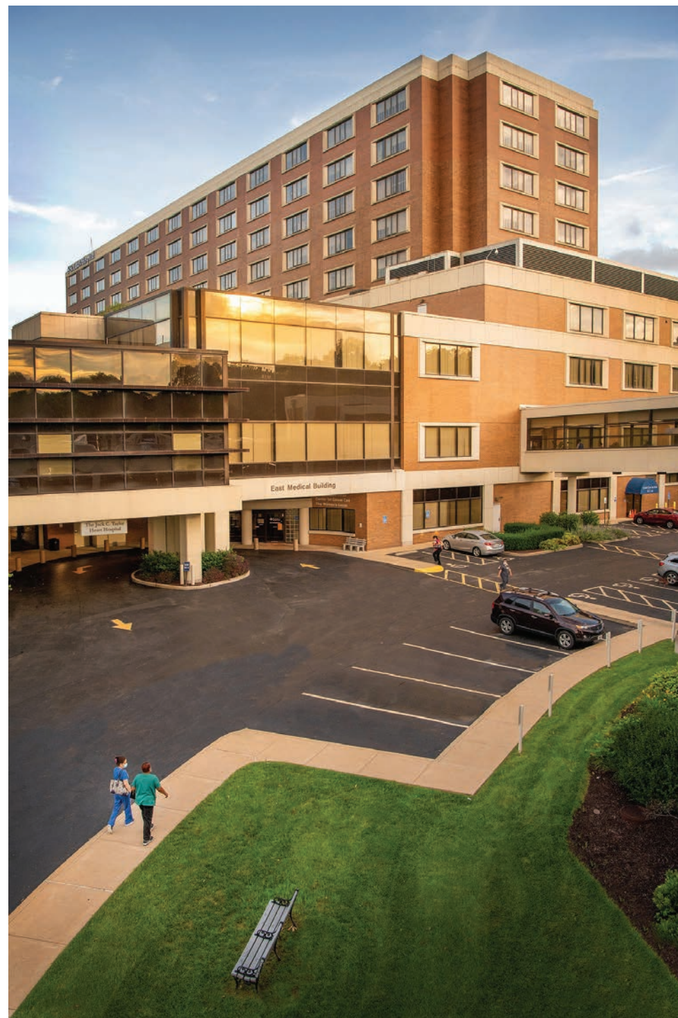
Jack C. Taylor Heart Hospital - East Medical Building
